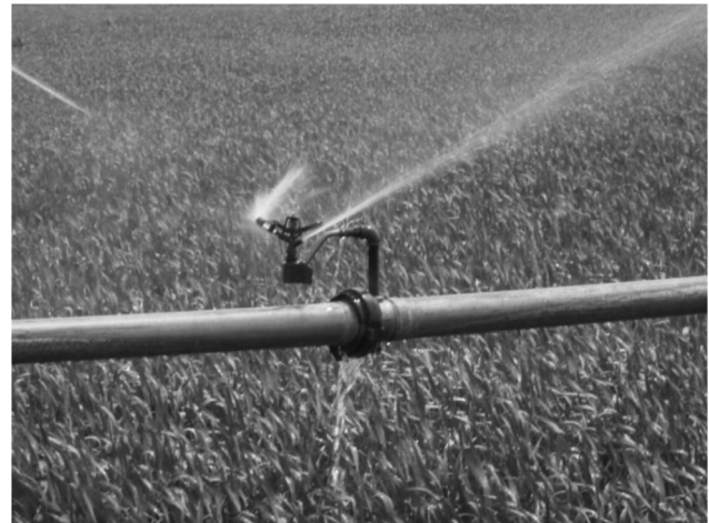
Figure 4. Water leakage from wheel move sprinklers
